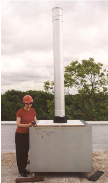
Figure 4 Light pipe under test on roof
